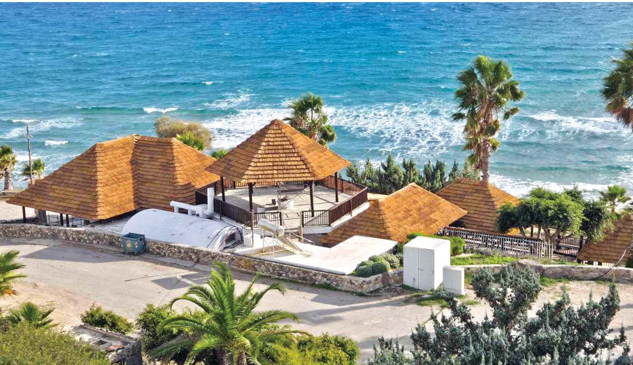
ΕΙΔΙΚΗ ΚΑΤΑΣΚΕΥΗ THATCH, PARASIDE BEACH ΚΩΣ - THATCHED CUSTOM CONSTRUCTION, PARASIDE BEACH KOS
