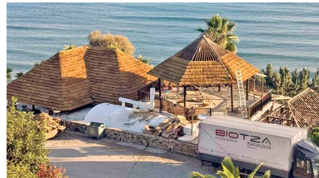
ΕΙΔΙΚΗ ΚΑΤΑΣΚΕΥΗ THATCH, PARASIDE BEACH ΚΩΣ - THATCHED CUSTOM CONSTRUCTION, PARASIDE BEACH KOS
